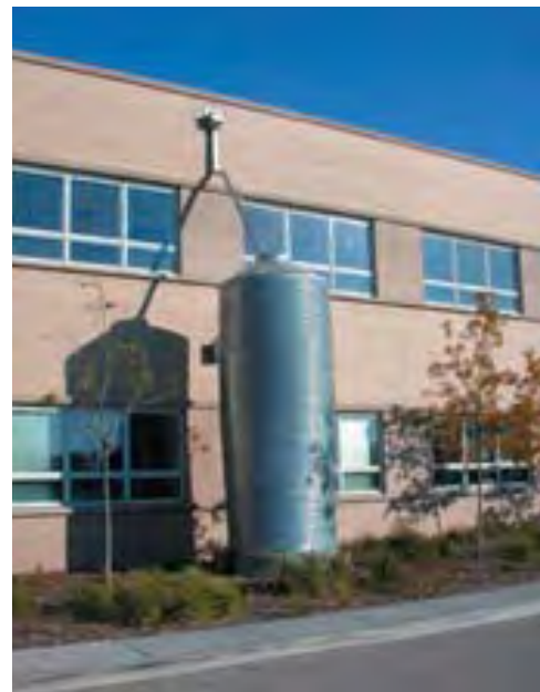
a cistern system collects rainwater from Chicago Center for Green Technology (Chicago, IL) (Photo: Conservation Design Forum)
